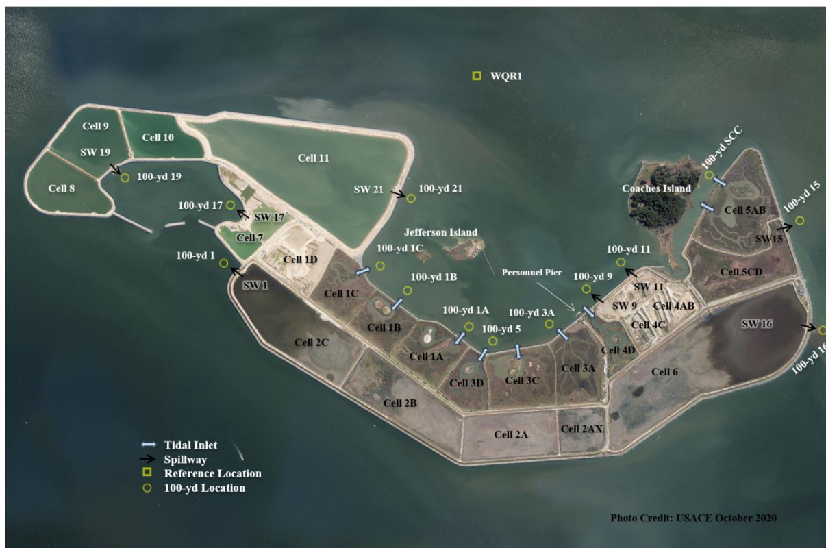
Figure 1. Paul S. Sarbanes Ecosystem Restoration Project at Poplar Island
